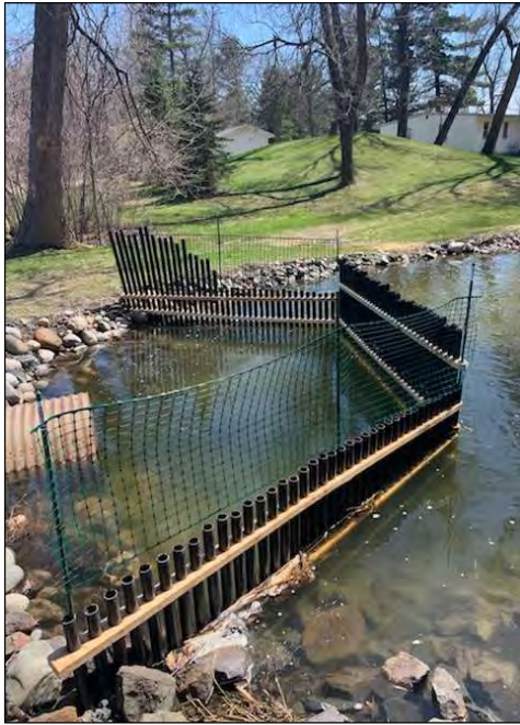
Left: Temporary carp barrier at Linwood Lake outlet.
